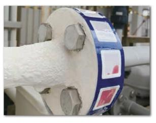
OIL DETECTION TAPE can be applied to areas at the risk of oil leaks, such as oil pipes of any oil encapsulation equipment (e.g., transformers, oil circuit breakers and condensers), flanges and valves.
